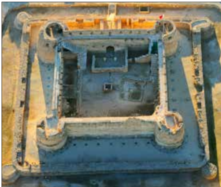
■ An aerial view of the Arad Fort
